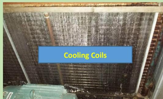
**Mold in Growing Room HVAC system Cooling Coil**
