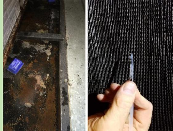
Mold on HVAC Cooling Coil Compartment & Coils
