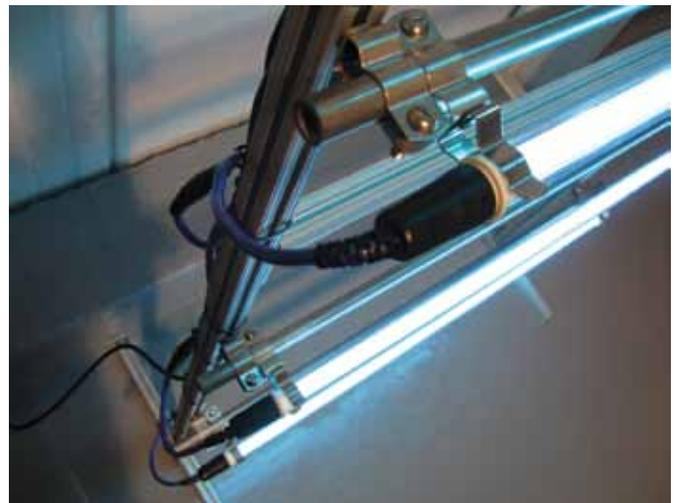
⚡ An important factor in a UVGI system is choosing a non-ballast model with a remote-power supply. A ballast and/or power supply has a shorter lifecycle when mounted in the humid corrosive environment of an air handler. In this photo, the single-pin UV lamps are connected to a remote-power supply via marine-grade, water-resistant connections.
