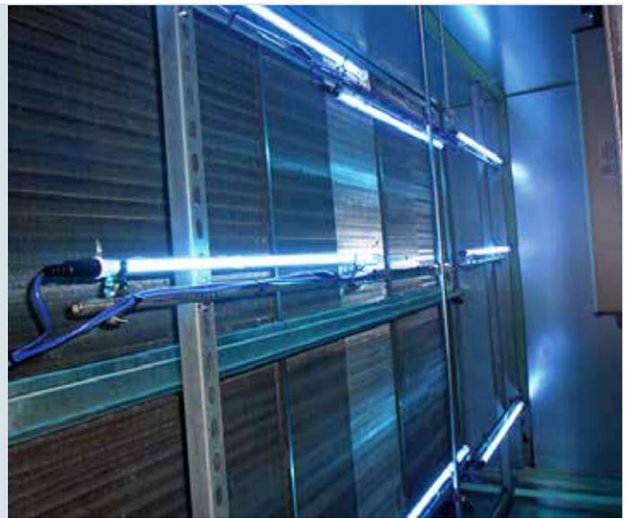
*UVGI is effective for microbial disinfection of interior wall surfaces, coils and the supply airstream of air handlers*
